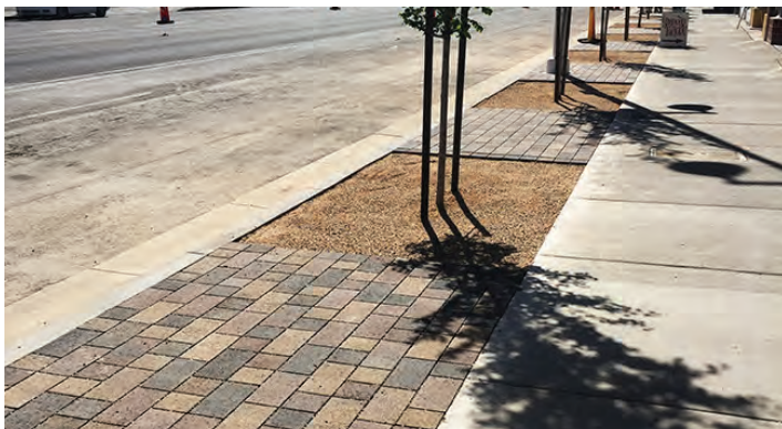
SIDEWALK WITH PERMEABLE PAVERS WITH TREES & PLANTING
