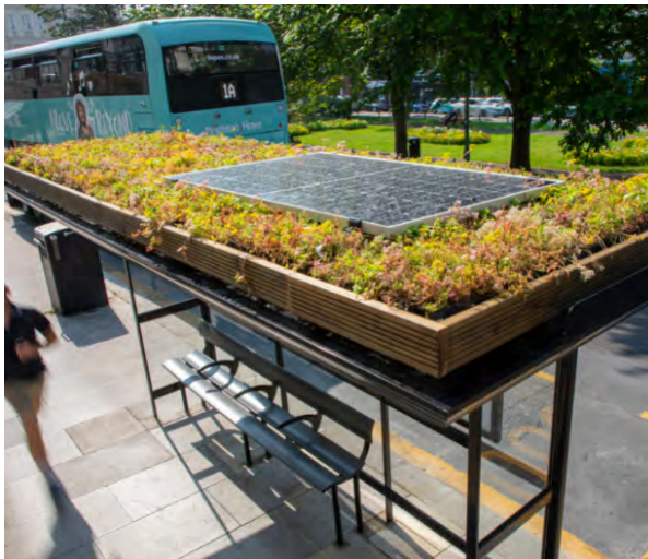
Green roof and solar panel to charge power source
