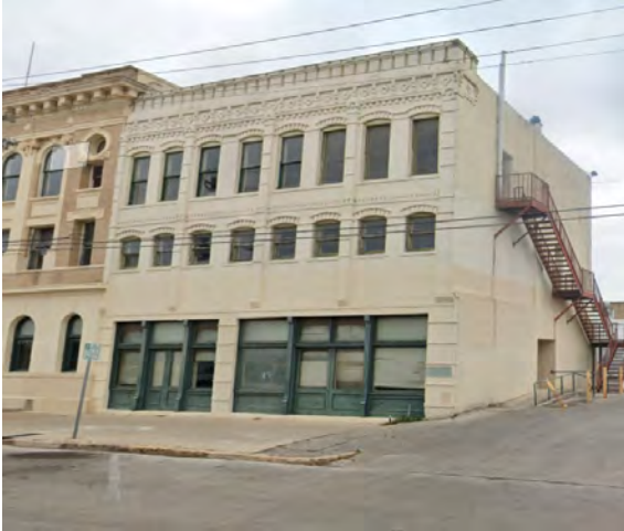
Existing building today
