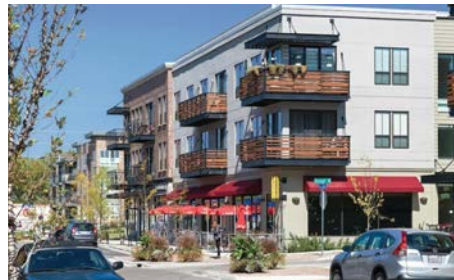
Infill of parking lots with street-facing mixed-use buildings
